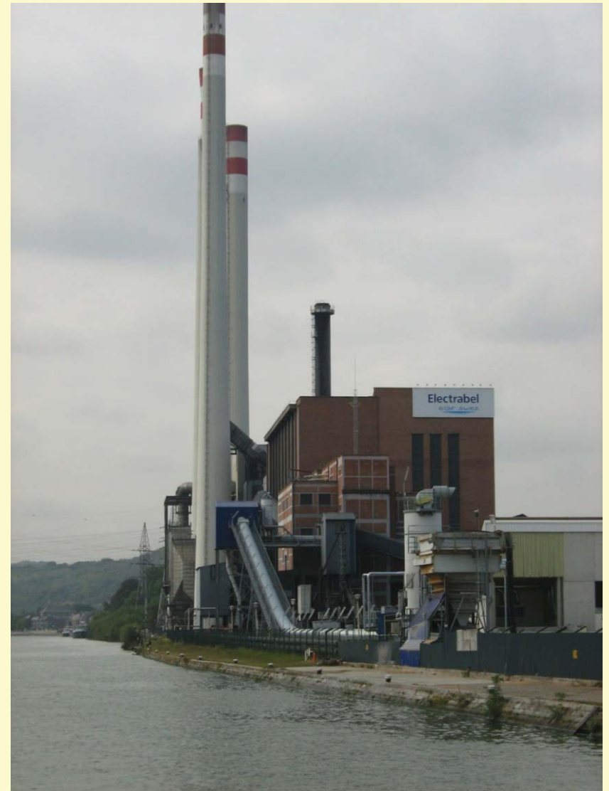
Les Awirs – converted from coal to pellets
