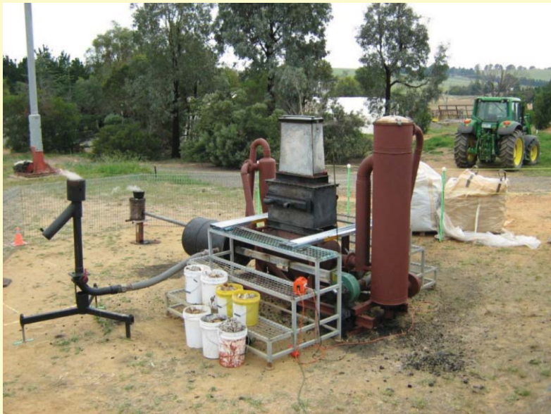
Real Power Solutions
