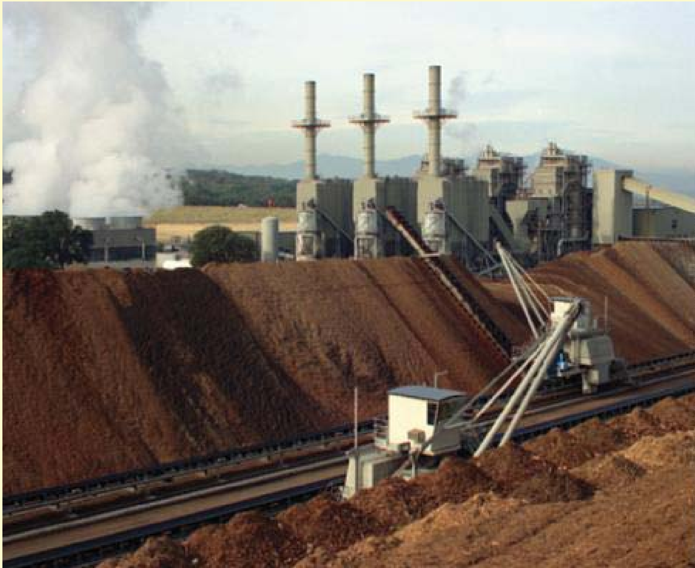
Shastra Anderson Plant (50 MW) – California
