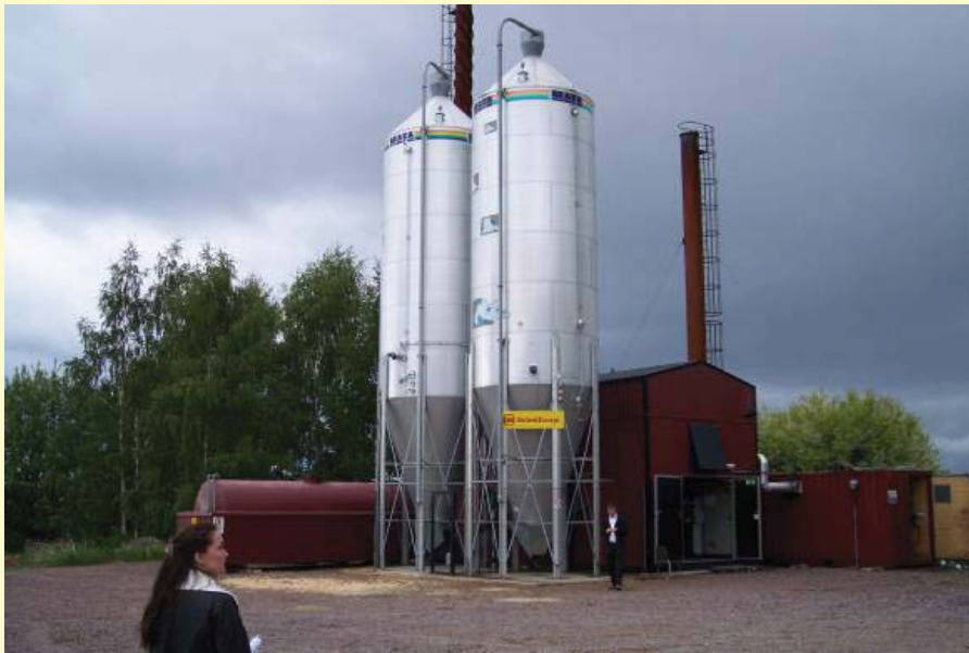
District heating plant
