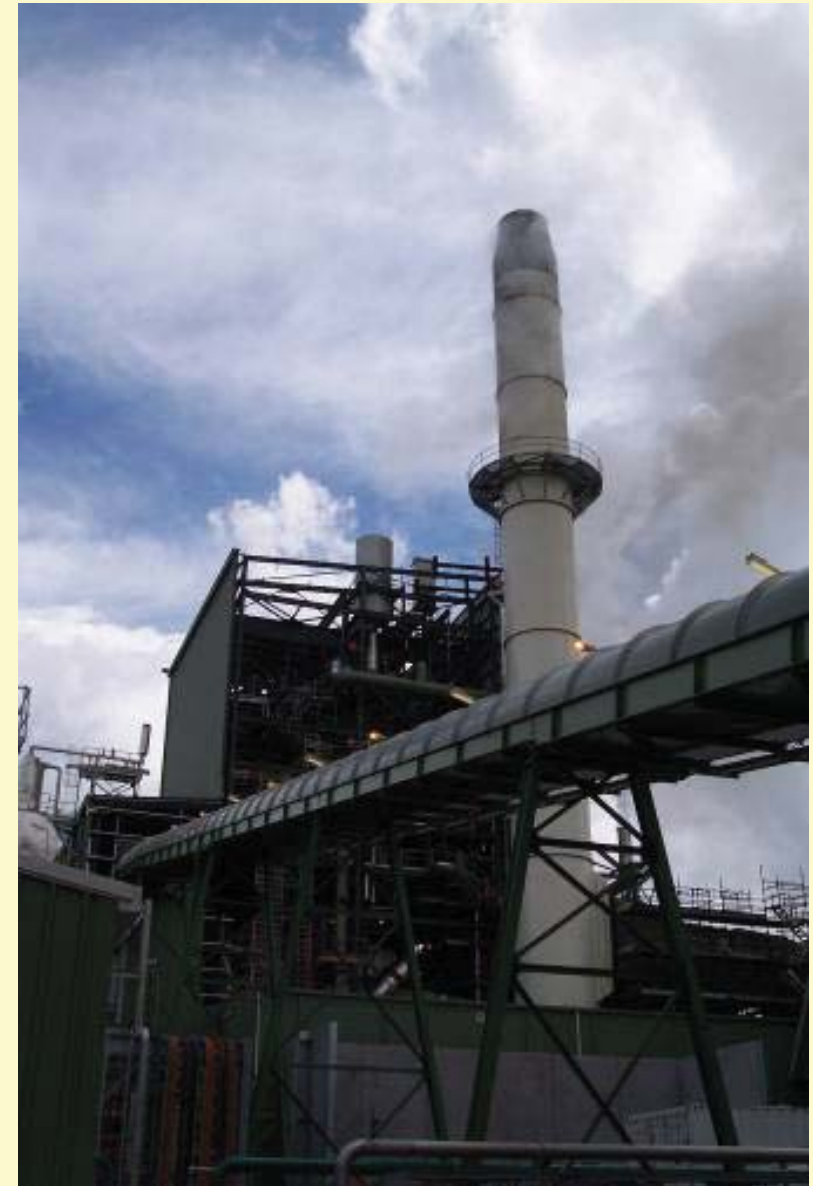
Condong Sugar Mill – NSW - 30 MW
